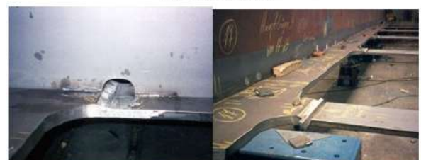
Fig. 14. The fillet welds holding this cover plate to the beam.
